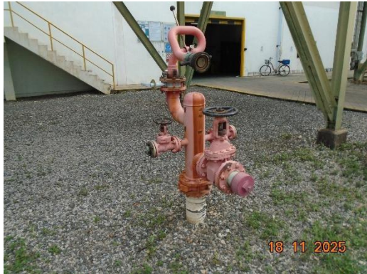
Water Hydrant/Fix Monitor
